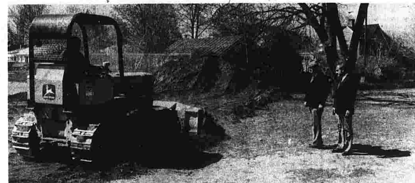
Playground work at Nathan Hale
